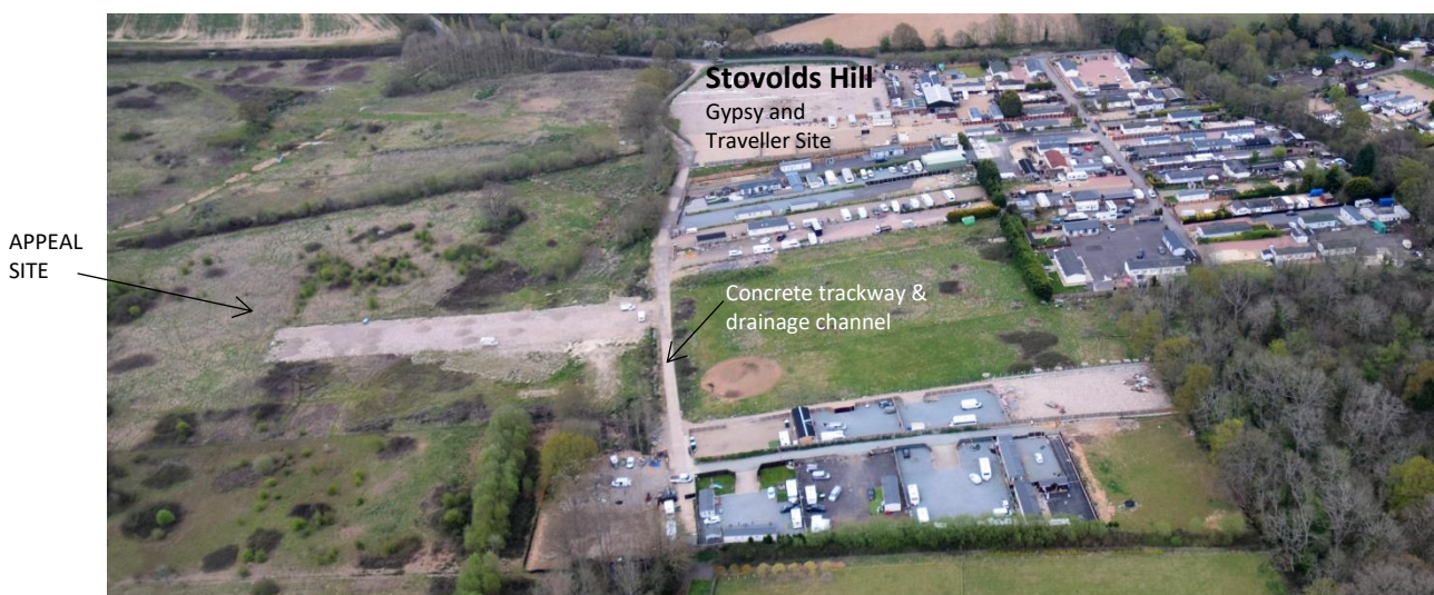
Figure 1: Gypsy and Traveller site showing the spread onto both sides of the concrete trackway, removal of a mature tree line and covering over of the drainage channel in 2022.
