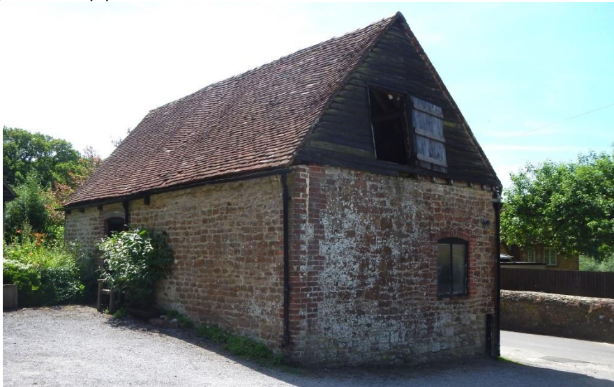
White Horse – stone barn with cast iron guttering and downpipes
